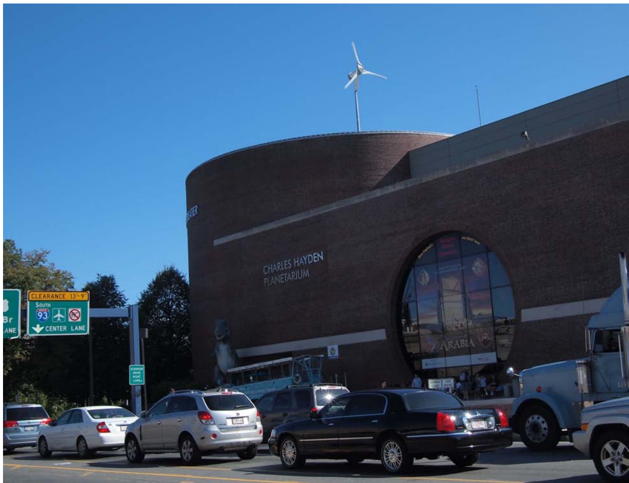
Boston Museum of Science showing one of many windmills on the roof.
